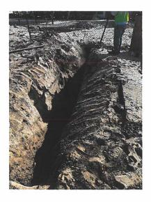
After ABS pipe was connected to the main line, they proceeded to pour road base gravel for compaction with the help of the compactor. Also, they replace the asphalt with new.
